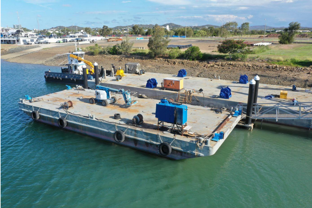
Figure 3.1 Flat-top barge ( https://www.fodico.com.au/wb3/ )
