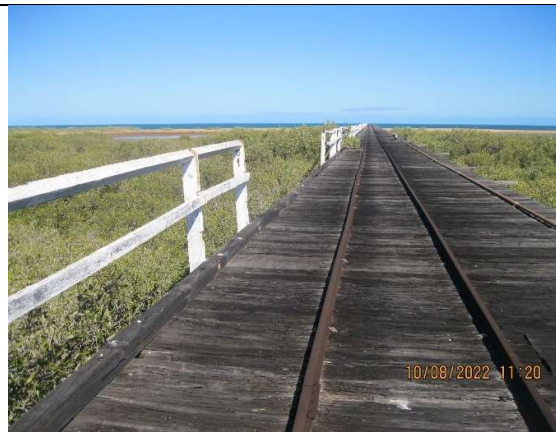
Photo 27: Missing handrailing
